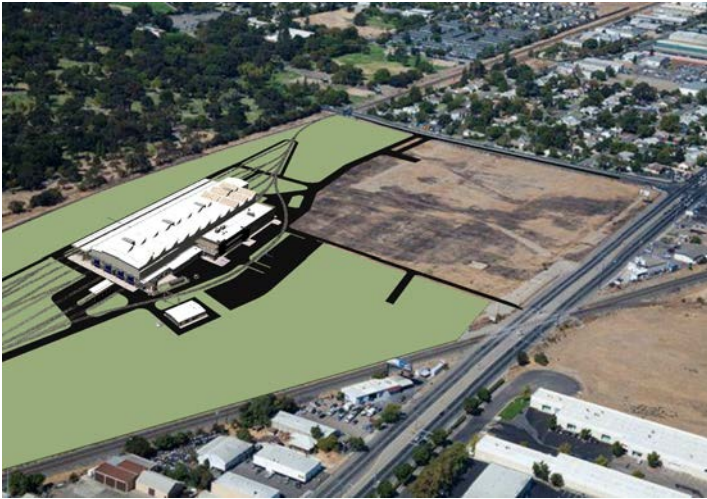
ACE Equipment Maintenance and Layover Facility
