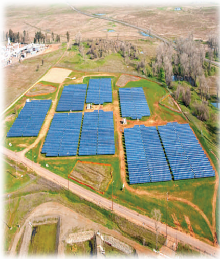
Solar Power Inc. solar farm.
