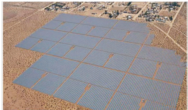
Pine Tree Solar Facility
