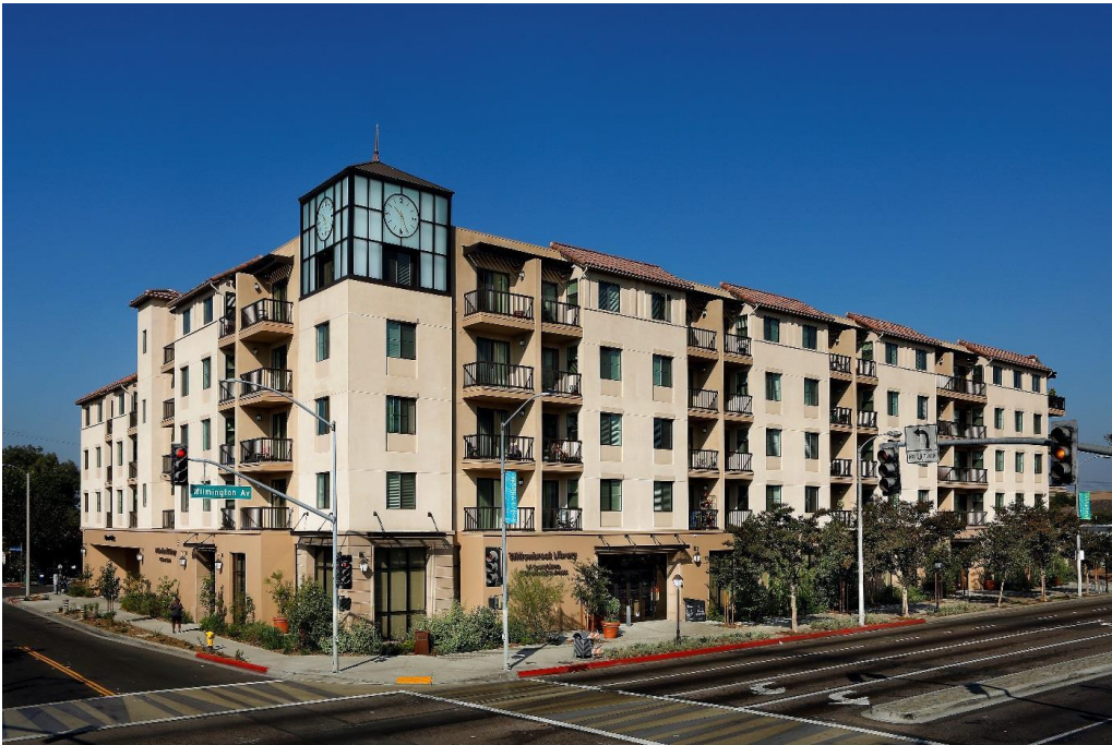
Project 16-002 in Los Angeles features community rooms, patio space and more for its residents.
