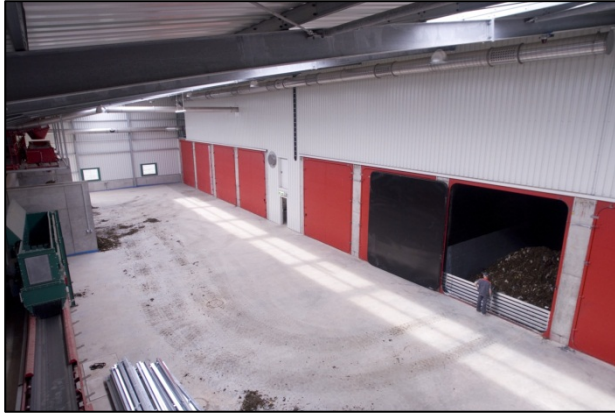
Mixing Hall and Anaerobic Digestion Tunnels
