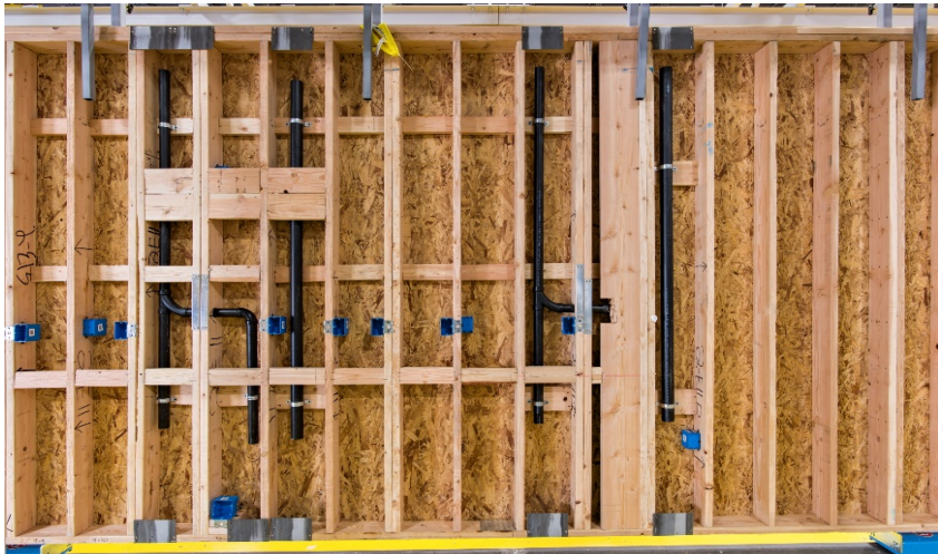
Figure 2: Example of an open wall panel constructed at Katerra’s factory before being shipped to the job site for assembly
