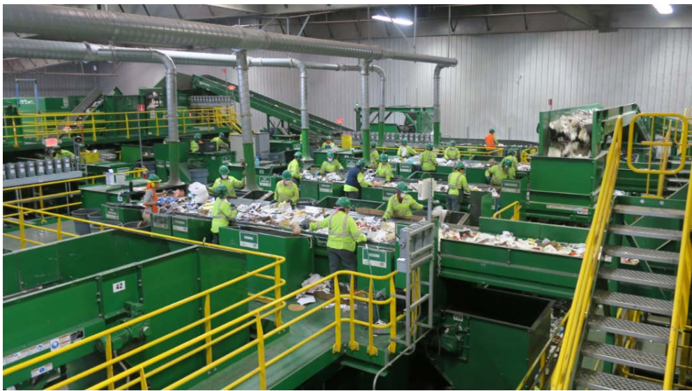
Figure 1: GreenWaste’s Materials Recovery Facility
