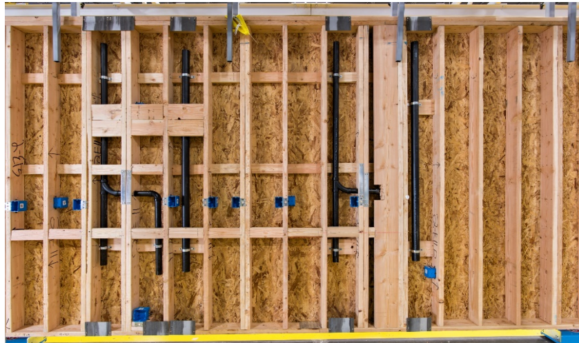
Figure 2: Example of an open wall panel constructed at Katerra's factory before being shipped to the job site for assembly
