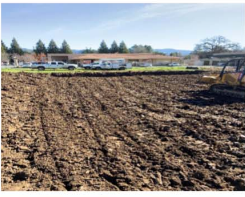
Bulldozer ripping the soil to air out and dry.
