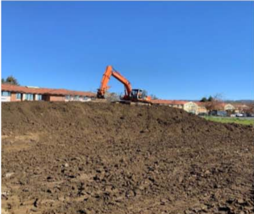
Excavator digging up dirt.
