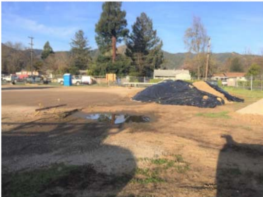
Stockpiled dirt material for driveway.
