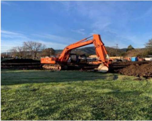
Excavator removing vegetation.
