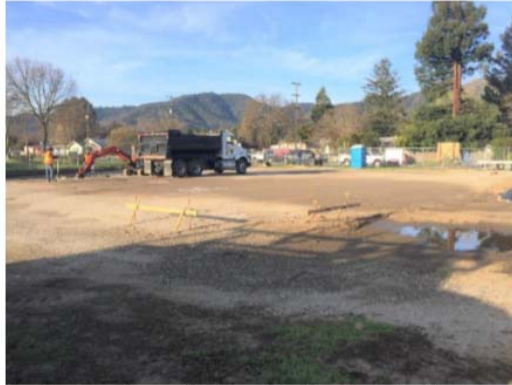
Batter boards used to layout footing lines for digging.
