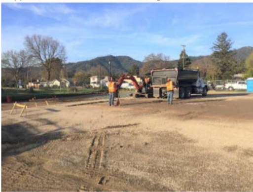
Cupples & Sons Const. crew working at south footing.
