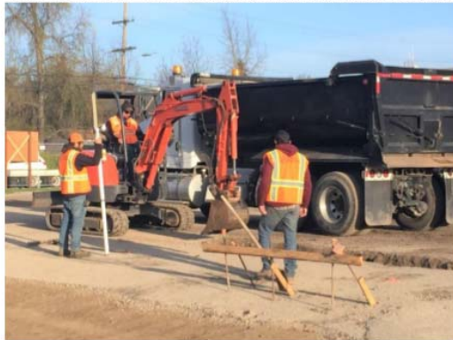
Footing depth checked with surveyor rod.
