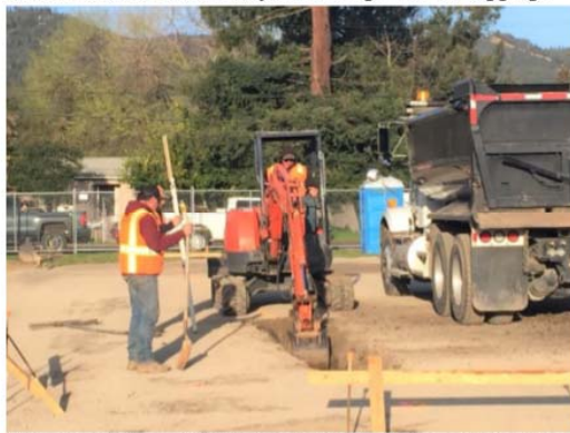
Cupples & Sons Const. digging & placing spoils in truck.
