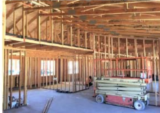
Open space area with vaulted ceiling framed.
