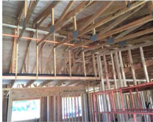
Fire sprinkler pipe above vaulted ceiling.
