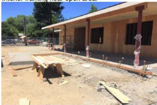
Front entrance concrete work and steel posts.
