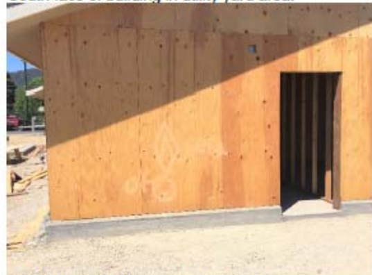
East face of building in utility yard area.
