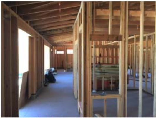
Interior framing at rear patio door.
