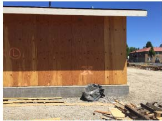
South face of building in utility yard area.
