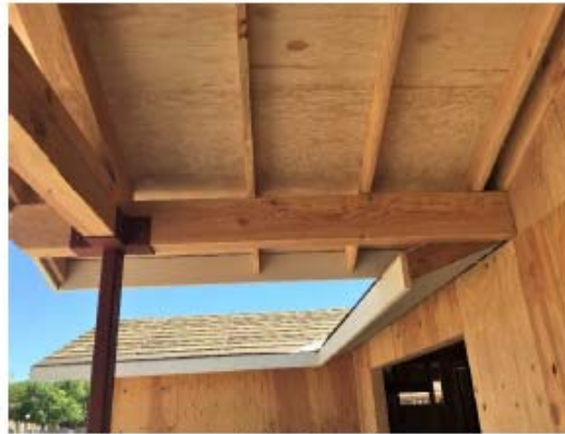
Open ceiling at exterior back patio area.
