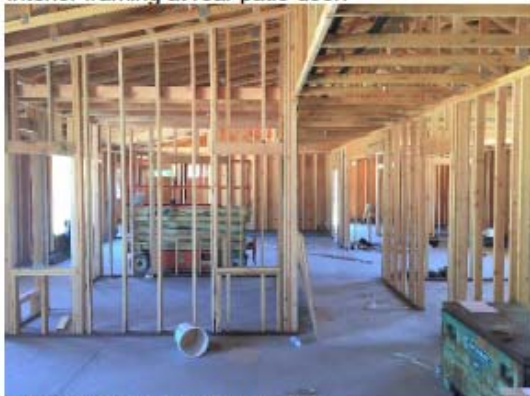
Interior framing near open area.
