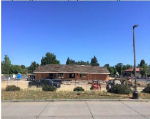
South face of building from Post Office parking lot.
