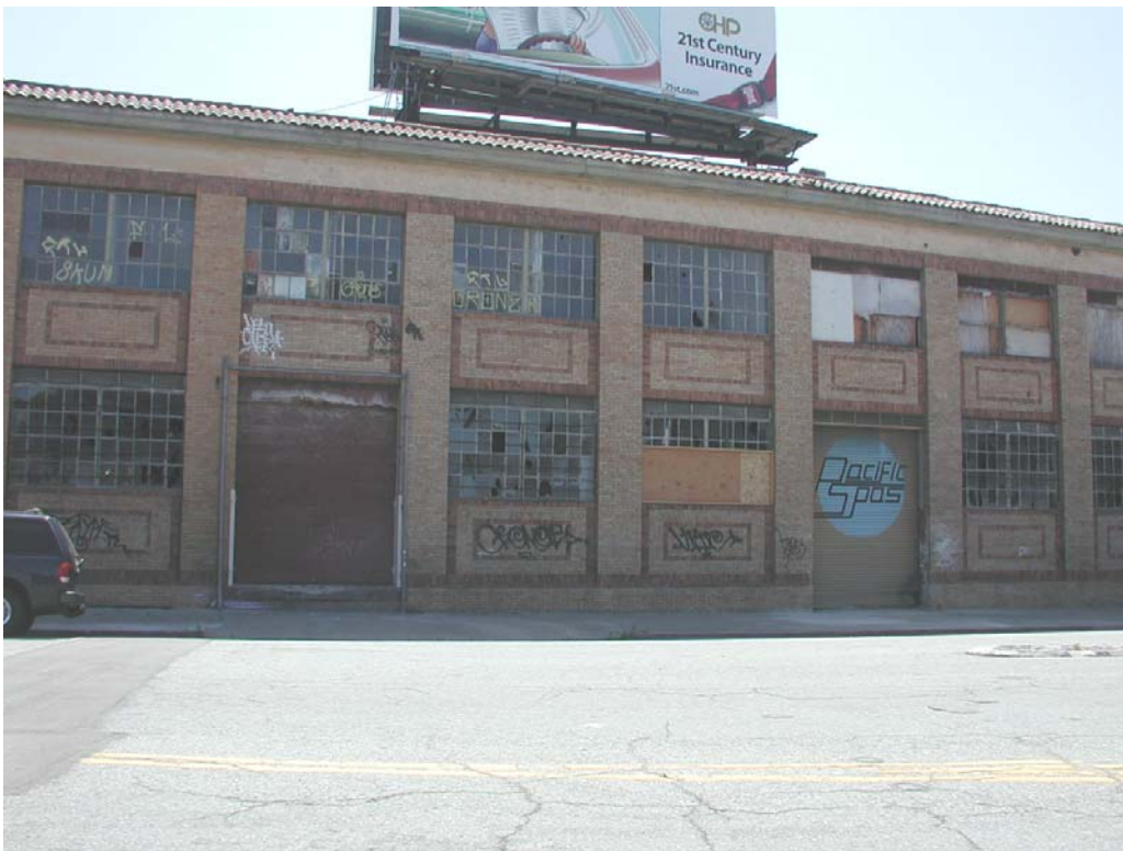
Project site before
