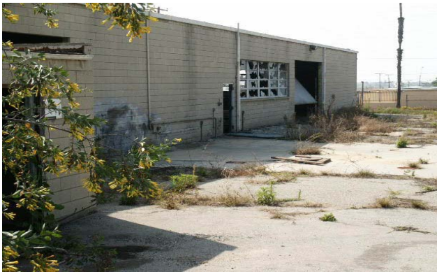
Project site before
