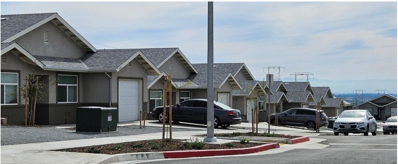
Brentwood Crossing in Bakersfield received state farmworker tax credits in 2022, as well as federal 4% LIHTCs, and will provide detached single-family rental homes for qualified domestic farmworkers. Brentwood Crossing is all-electric and provides an on-site manager's home, community center, and playground and broke ground and opened in 2023.
